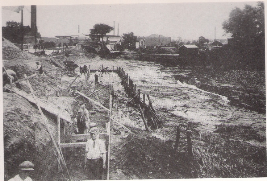
74. Harborne Lane (July 10th, 1929). These men would seem to be rebuilding the side of the Dudley canal. This photograph was taken from the footbridge at the Harborne Lane entrance to Selly Oak Park looking south towards the Bristol Road.
