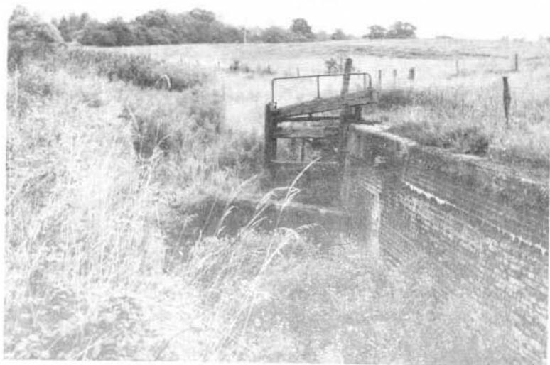
Lock 4: Again a chamber clearance. The channel above and below will be cleared by a large excavator.
