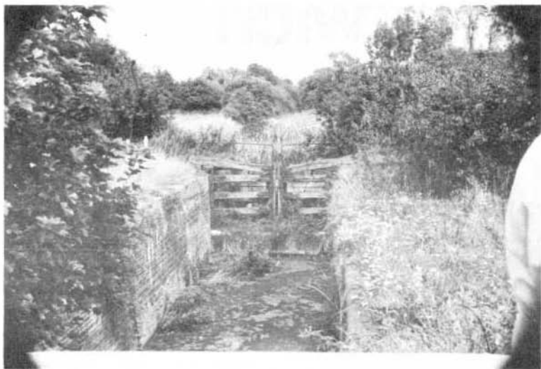
Ladywood Top Lock: Chamber clearance - a drainage channel is to be dug and the brickwork repaired.
